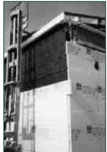
Figure 2: Conventional dampproofing and insulation.
