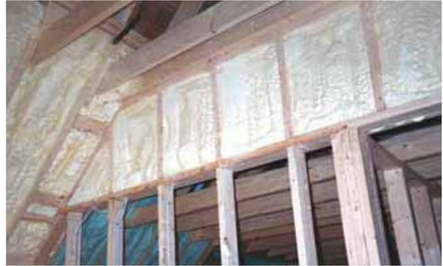
According to the National Association of Home Builders Research Center, a structure braced with SPF-filled walls suffers less damage and permanent deformation of wall elements during a hurricane.
